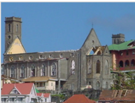
Hurricane-church roof gone
