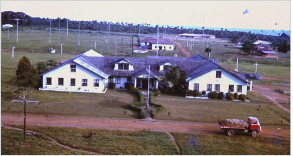
ELWA studio building in foreground, transmitter building behind studio, hospital in the background, Academy to the right, homes along the Atlantic Ocean
