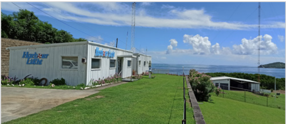
Studio & office buildings completed
