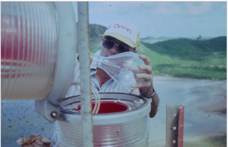
Rolen replacing the light at the top of the tower
